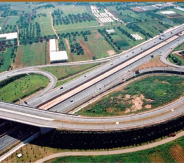
Aerial View of the Attiki Odos Motorway
