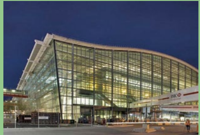
Heathrow Airport's T5 Terminal
