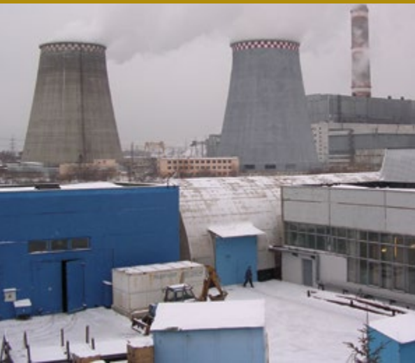
Main Plant at Mosenergo Heating and Pipeline Moscow, Russia
