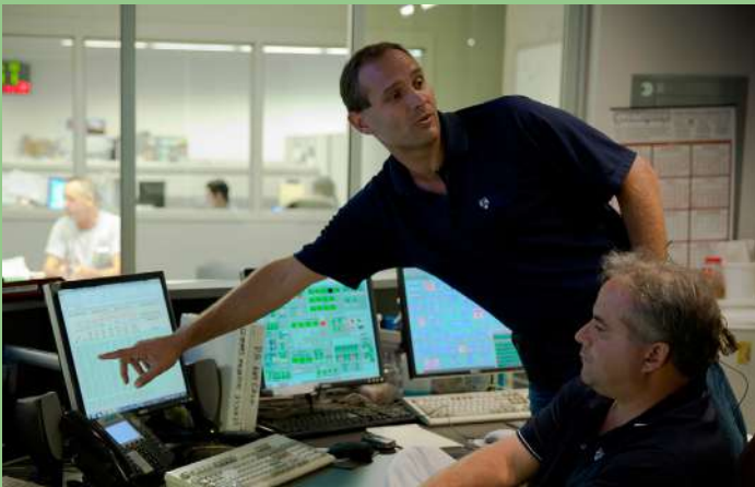
Penn's Operational Control Center (OCC) running ICONICS GENESIS64™
