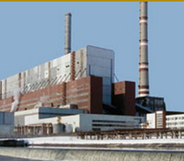
Permskaya Gres Power Plant Dobryanka, Russia
